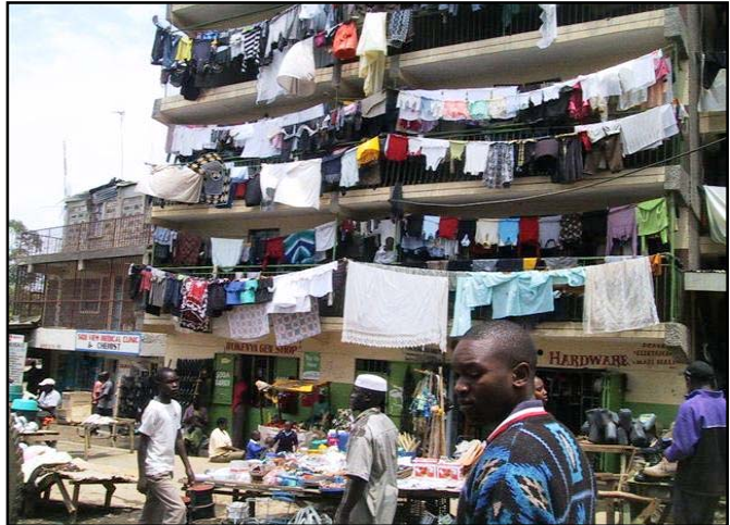
Outside of the WEEP center on main drag.
